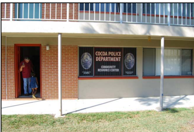
The Cocoa Police Department substation at 800 N. Fiske Blvd. doubles as a Community Resource Center.
